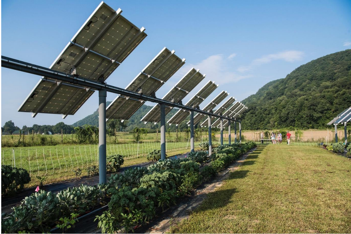
Picture7: Vegies under the shade of PVs, the morning moist condensates at the PVs improve the water availability, while the evapotranspiration of the cover crop reduces heat. Photo: UMASS NREL
